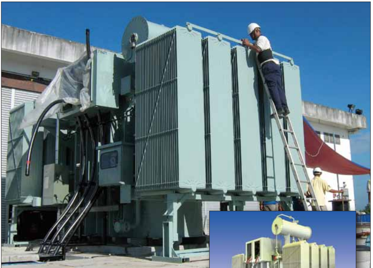
• Power Transformer on site installation
